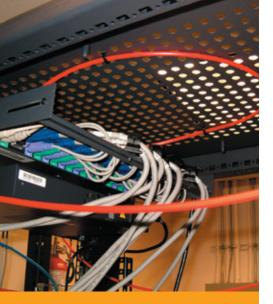
Firetrace does not occupy valuable rack space. This red Firetrace Detection Tubing can be run unobtrusively across the top of the rack.
